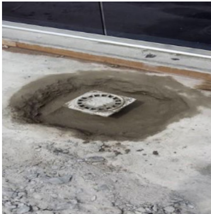
Elevator pit after waterproofing
