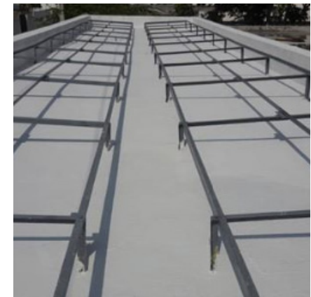
After waterproofing work
