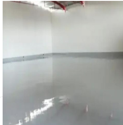
Epoxy Flooring System
