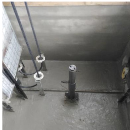
Walls after waterproofing
