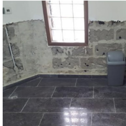
Damp Walls Treatment
