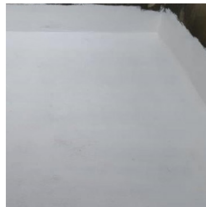
Overhead tank after waterproofing
