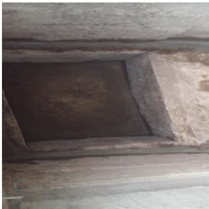
After waterproofing work
